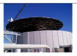
Installation of the geodesic dome covers, June 2011
