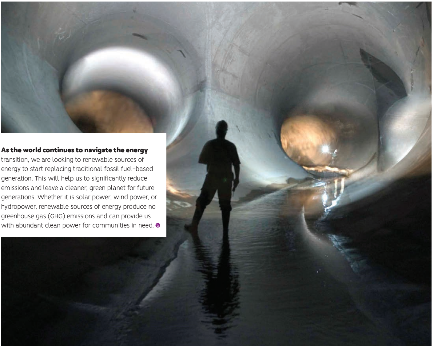
Above: Inspecting Rocky Mt pumped storage tunnels ALL IMAGES COURTESY OF STANTEC
