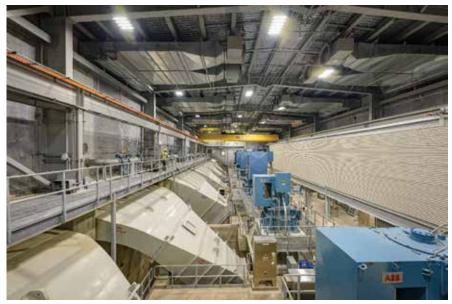
Figure 2: Interior of the 17th Street Pump Station showing its array of siphon discharge tubes and combination of blue vertical gear-motors: 2,500 HP motors for the 900 cfs pumps in the foreground and 5,000 HP motors driving the 1,800 cfs pumps in the background.
