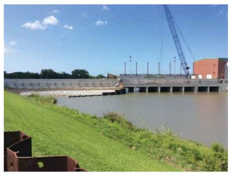
Figure 3: Bypass gate structure at London Avenue outfall canal site.
